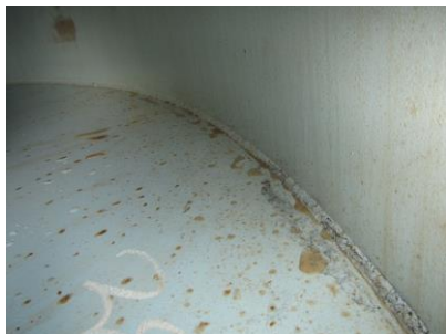
FLOOR TO SHELL WELD
