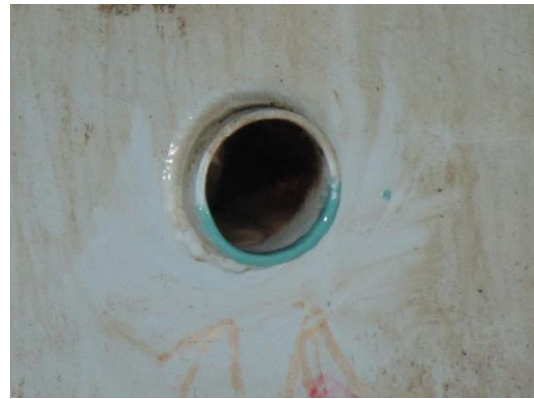
NOZZLE COATING REPAIR
