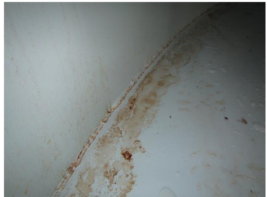
FLOOR TO SHELL FILLET WELD
