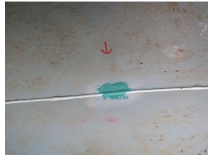
FLOOR LONGSEAM COATING REPAIR
